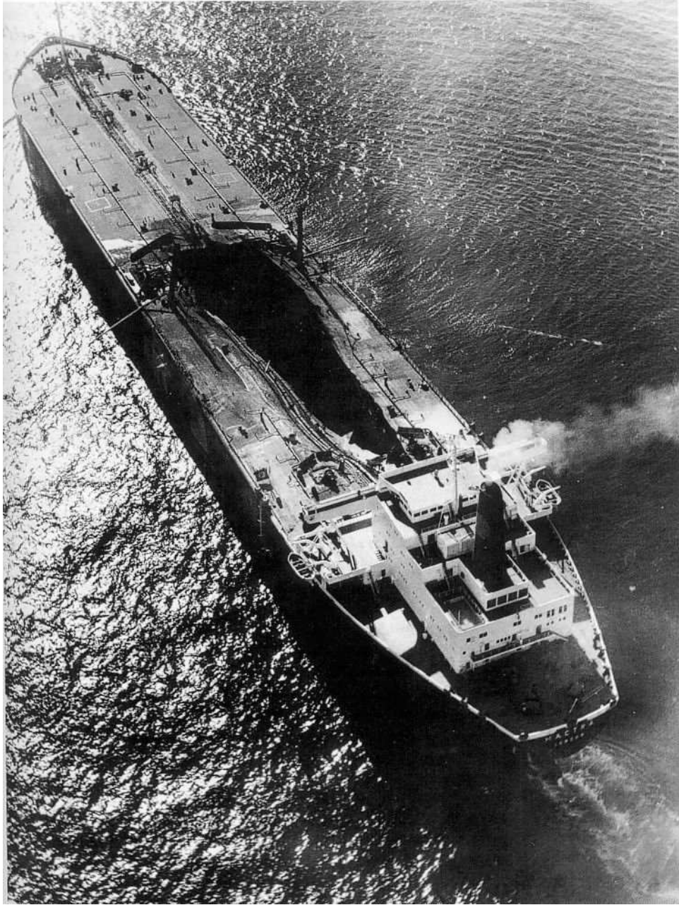
Figure 2: Mactra deck after tank cleaning explosion. Two killed. Source: Auke Visser, supertankers.topcities.com
